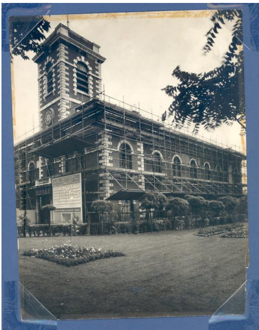
Left: The church under scaffolding During the post-war rebuilding 78
