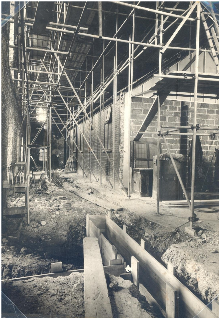
The temporary church built inside the bombed shell of the church 64
