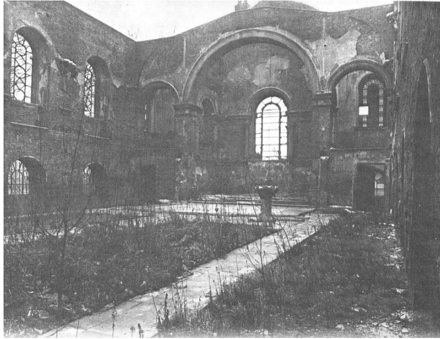
The interior of the bombed church (looking towards the north east) after clearing 55
